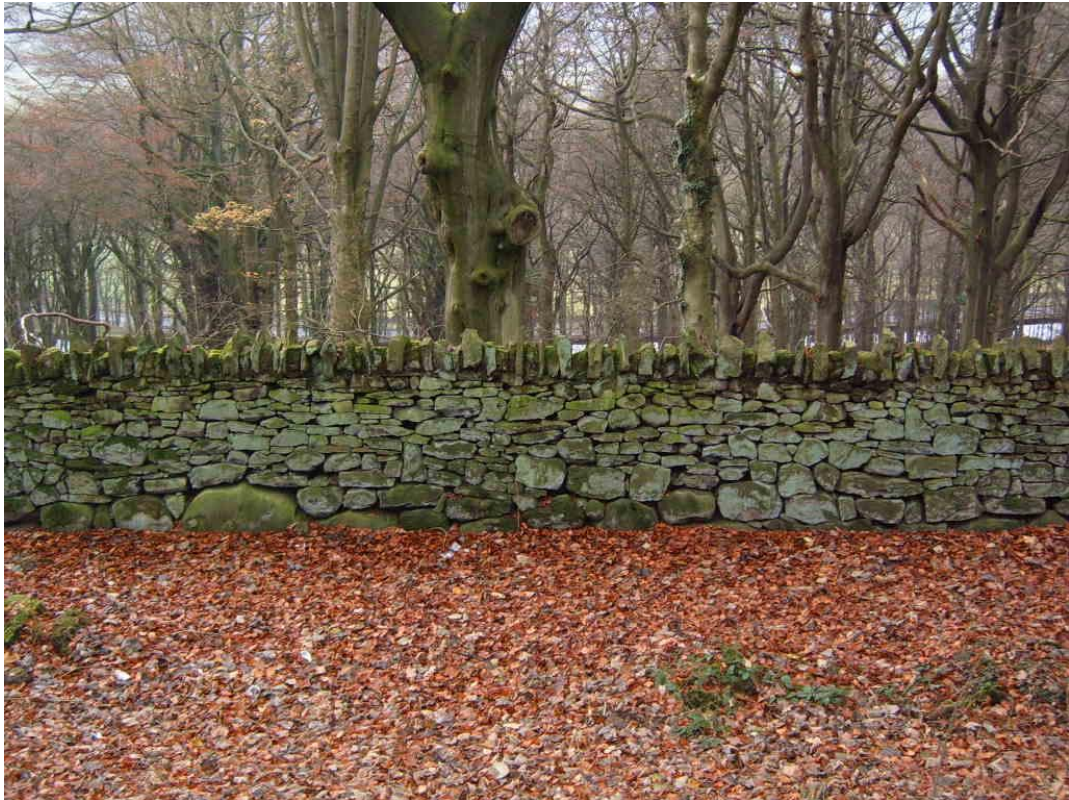
Fig 6: This and the previous photograph overlap to show a section of the Eastern wall, photographed from Bradley Lane, with an almost continuous stretch of orthostats at the base.
