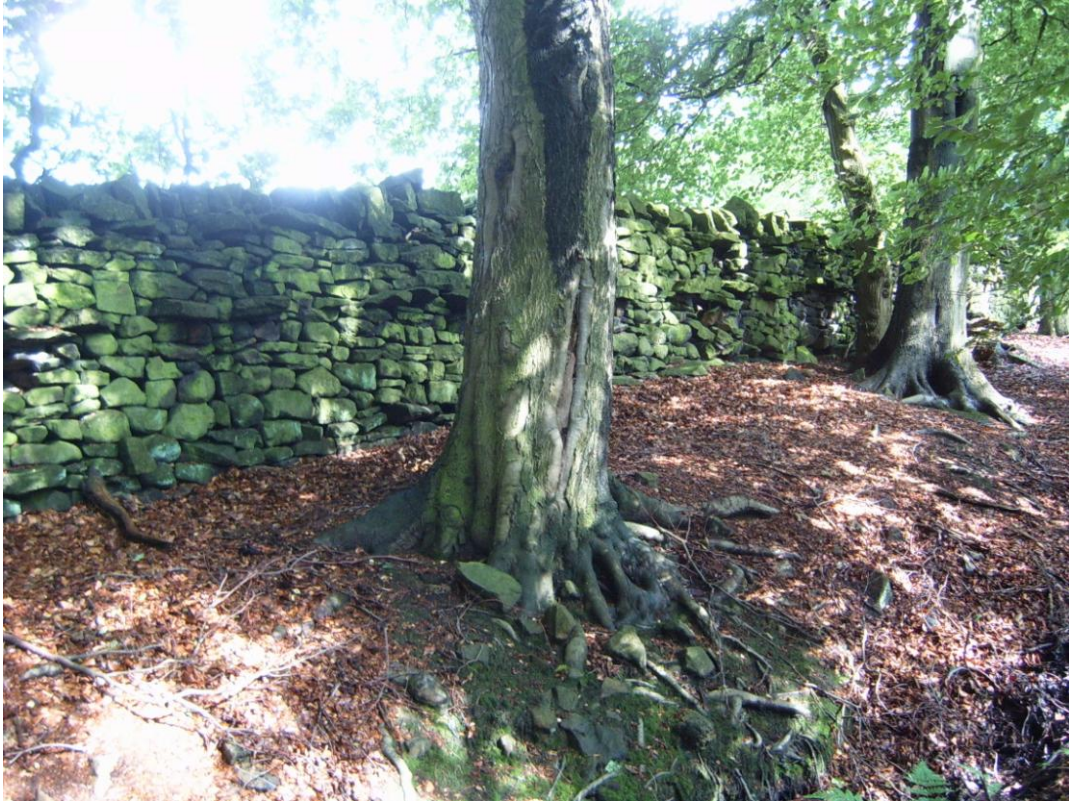
Fig 12: Part of the Northern (Bradley) boundary wall, photographed from within the wood. No orthostats are present and a single regular line of throughs has been used.
