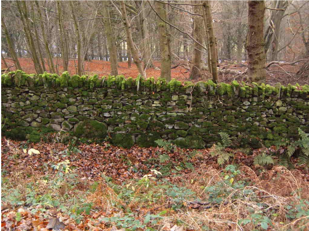
Fig 7: Another section of the Eastern wall, photographed from Bradley Lane. Again showing orthostats at the base.
